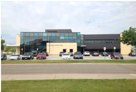
NDUS IT Office building.
